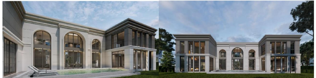
The Menara Hill – The Menara Resident Kamala
